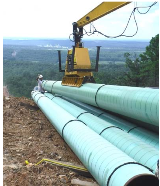
Positioning is very easy even with long and heavy pipes. 049-05-05-033A
